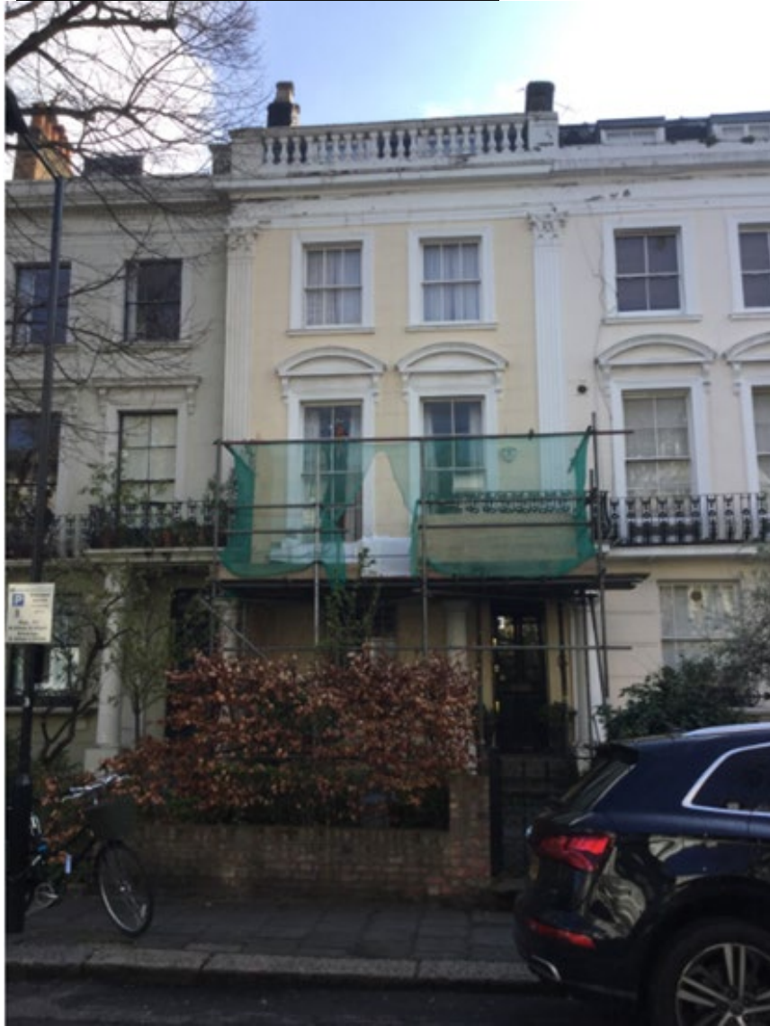
Front Elevation After Removal of Balcony
