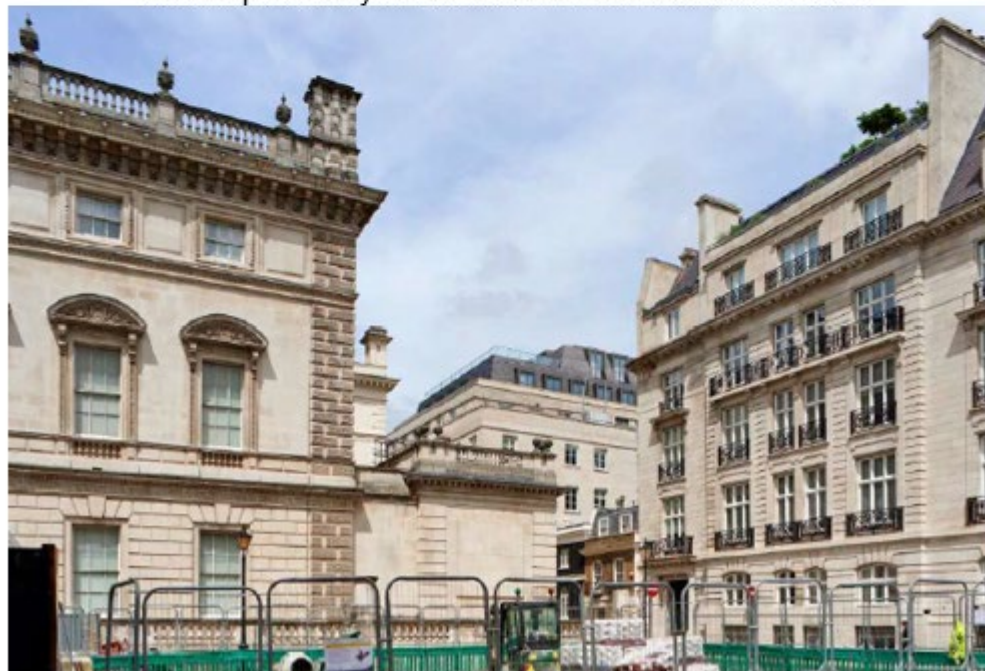
View of previously refused scheme from Cleveland Row
