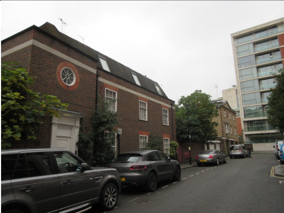
Site Prior to Demolition of the Buildings
